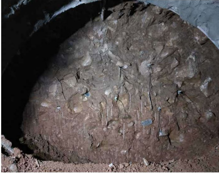
a) Bench excavation in headrace tunnel in clay with gravels
