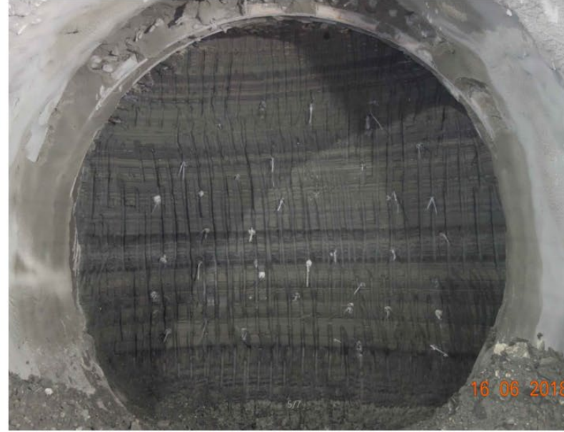
b) Full face excavation in tailrace tunnel in marl
