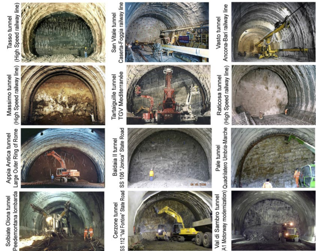
Fig. 2. Photographs showing the face of a few selected tunnels excavated full-face by using the "heavy method" (Lunardi and Barla, 2014).
